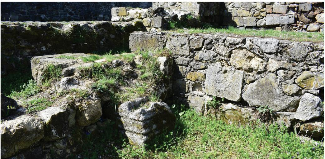
Figure 17 The foot of the pilaster carrying the cross vault of the church
