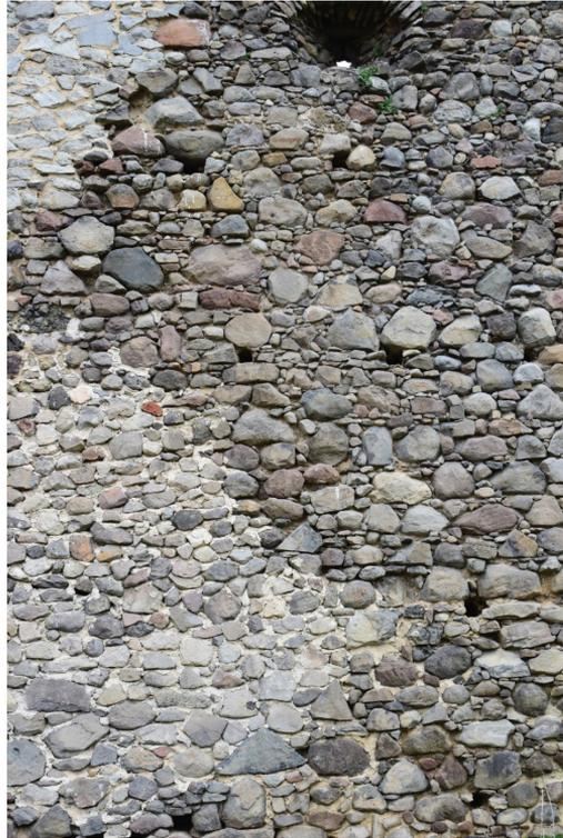
*Figure 38 Appropriately done reconstruction of the fortifications with new masonry distinguishable from the original*
