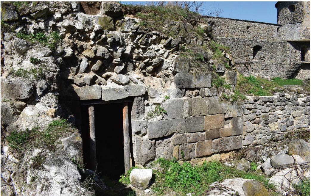
Figure 27 Block masonry with a core in a spiked weave in the northern towers of the monastery church
