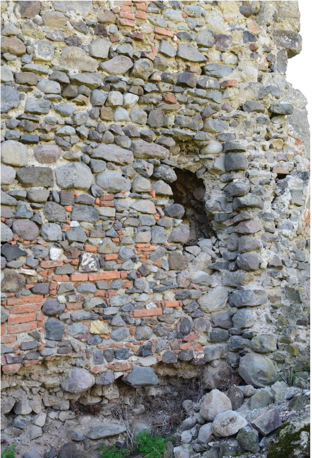
*Figure 29 Detail of mixed masonry*
