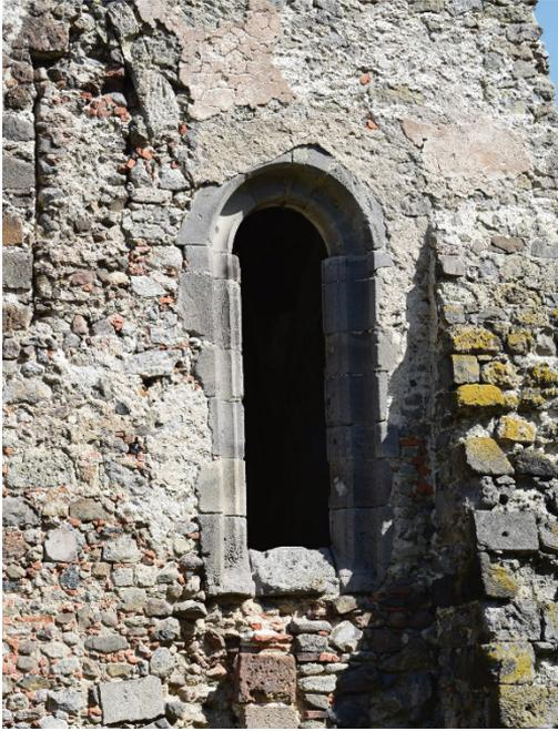
Figure 24 Gothic window with a tracery from the extinct church, secondarily reassembled during the conversion of the sacristy into a chapel
