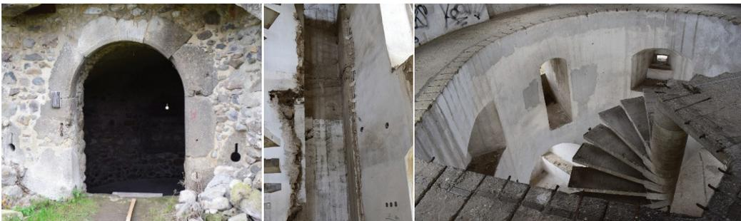
*Figure 37 Negatively affecting adaptation elements: a) incorrectly reconstructed details b) invasive installation of engineering networks, c) reversible communication elements*
