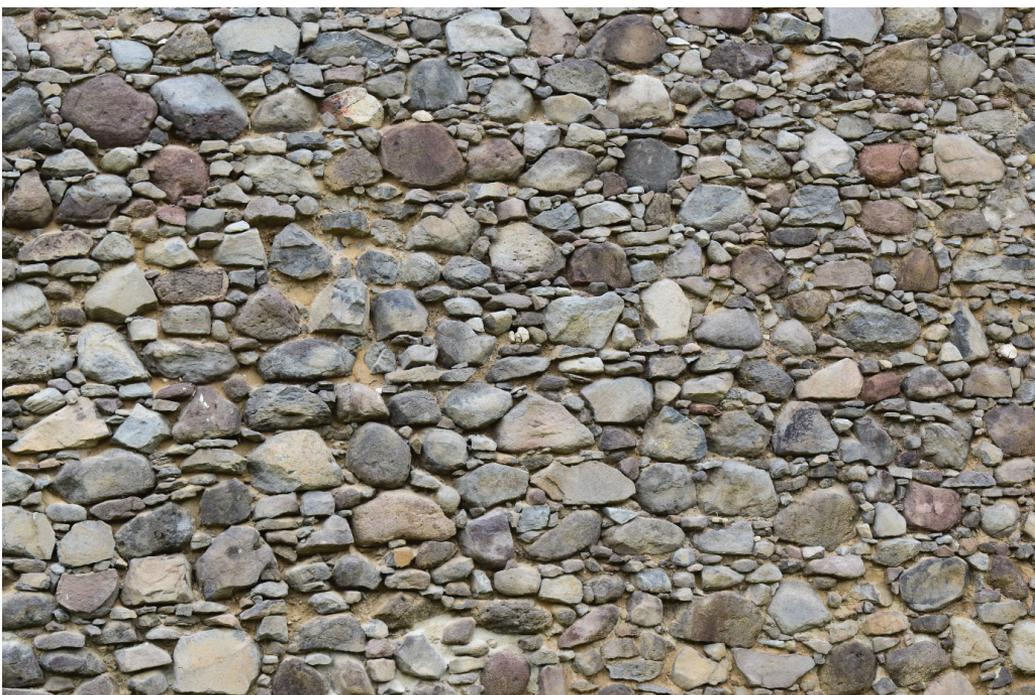
Figure 28 Rubble masonry – the most common type of building structure
